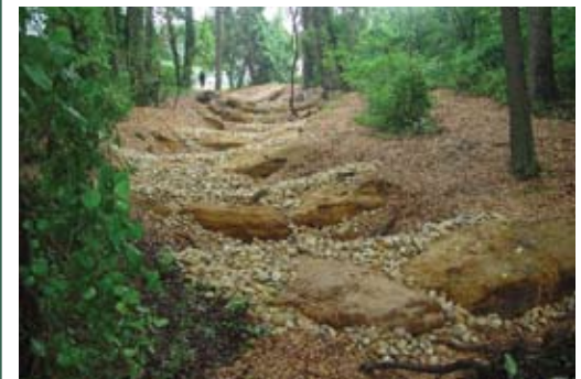
After Restoration - Dry Conditions Step Pool Storm Conveyance System
