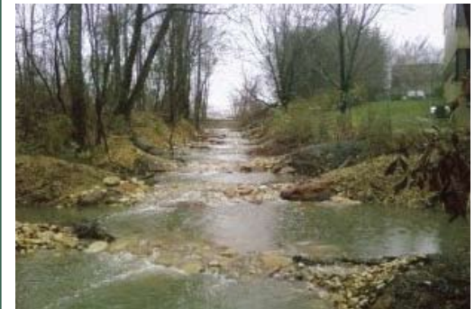
After Restoration - Wet Conditions Step Pool Storm Conveyance System
